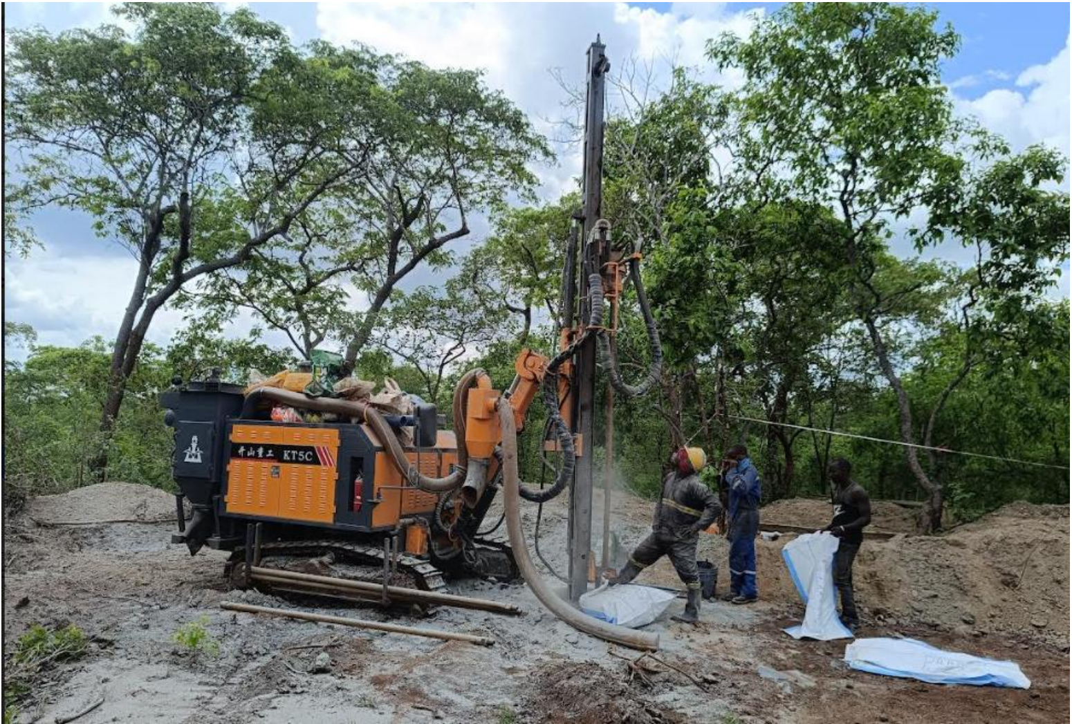
Reverse Circulation Drilling with 796 metres drilled in 18 holes drilled with a total of 1506 samples collected.
